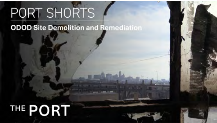
ODDO Site Demolition & Remediation | July 2023
