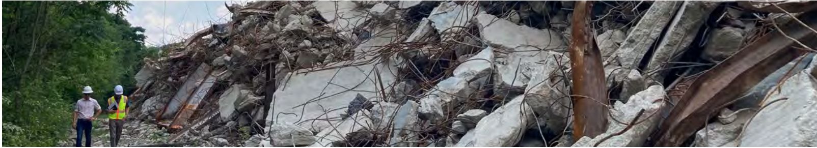
Beckman Silos Demolition | Millvale
